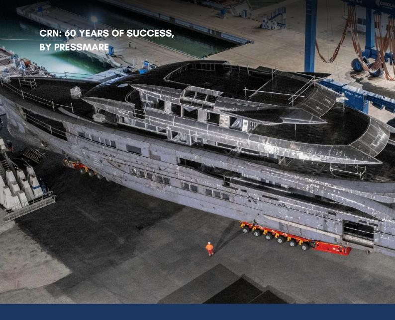
Investing in expanding the facilities at the Ancona hub has been a multi-stage process that continues to this day and has seen it develop into the Ferretti Group Superyacht Yard. Spanning 80,000 sqm (around 33,000 of which indoors), it can accommodate 24 superyachts and pleasure vessels under construction, from 30 to 90 metres in length.
